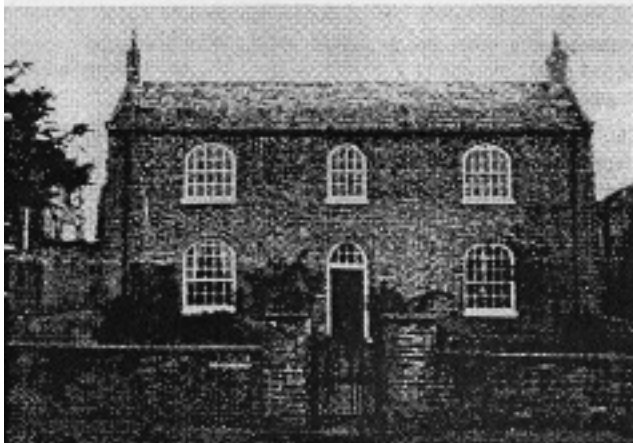
The Old Vicarage, Church Street
